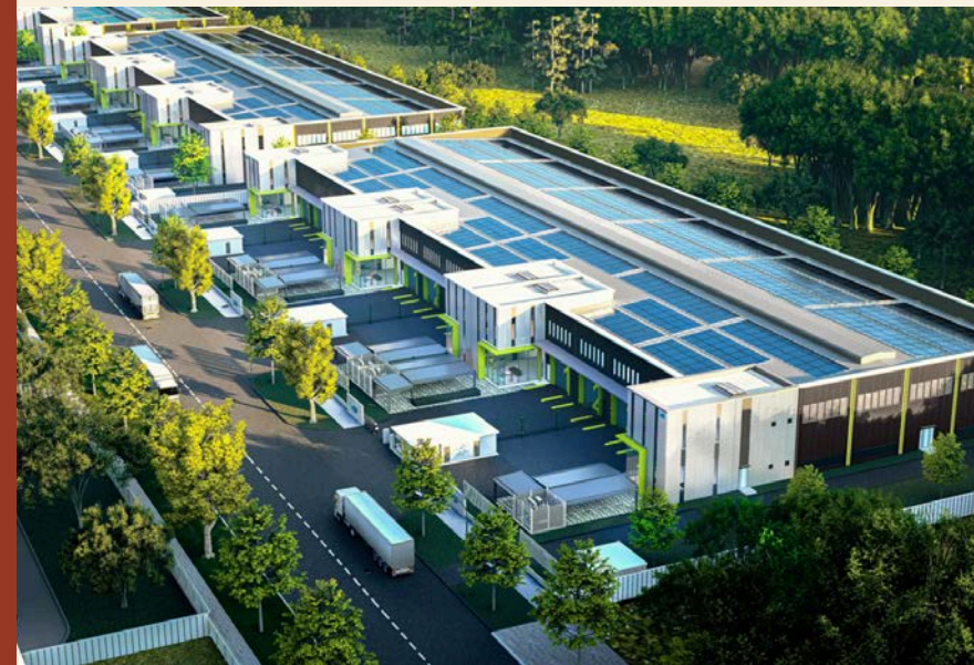
READY BUILD FACTORIES OF PHASE 2 AT VSIP III, HO CHI MINH CITY, VN
